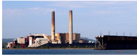
Presque Isle power plant
