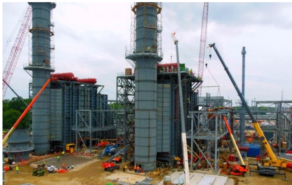
West Deptford Energy power plant construction | MJ Energy
