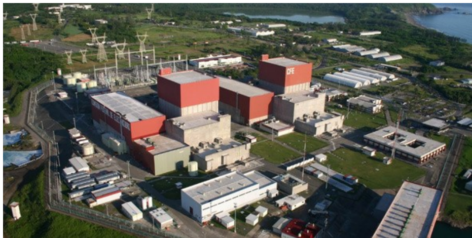
Laguna Verde, Mexico’s sole nuclear plant. It is owned by CFE, the state utility. | nuclear-energy.net
